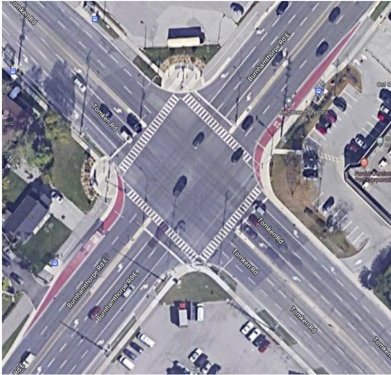
Figure 5: Far-side bus bays, Burnhamthorpe Road, Mississauga
