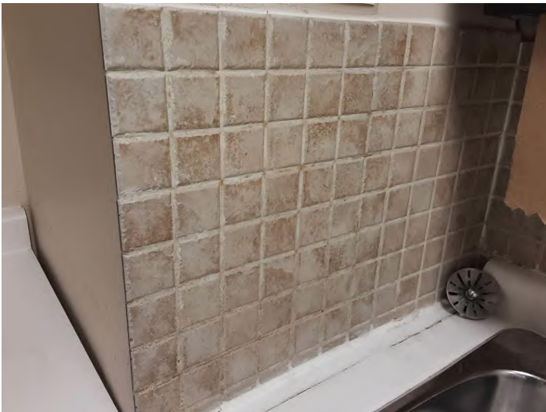
V0000 (None), Wall, Ceramic Tiles, Kitchenette (Location #: 81)
