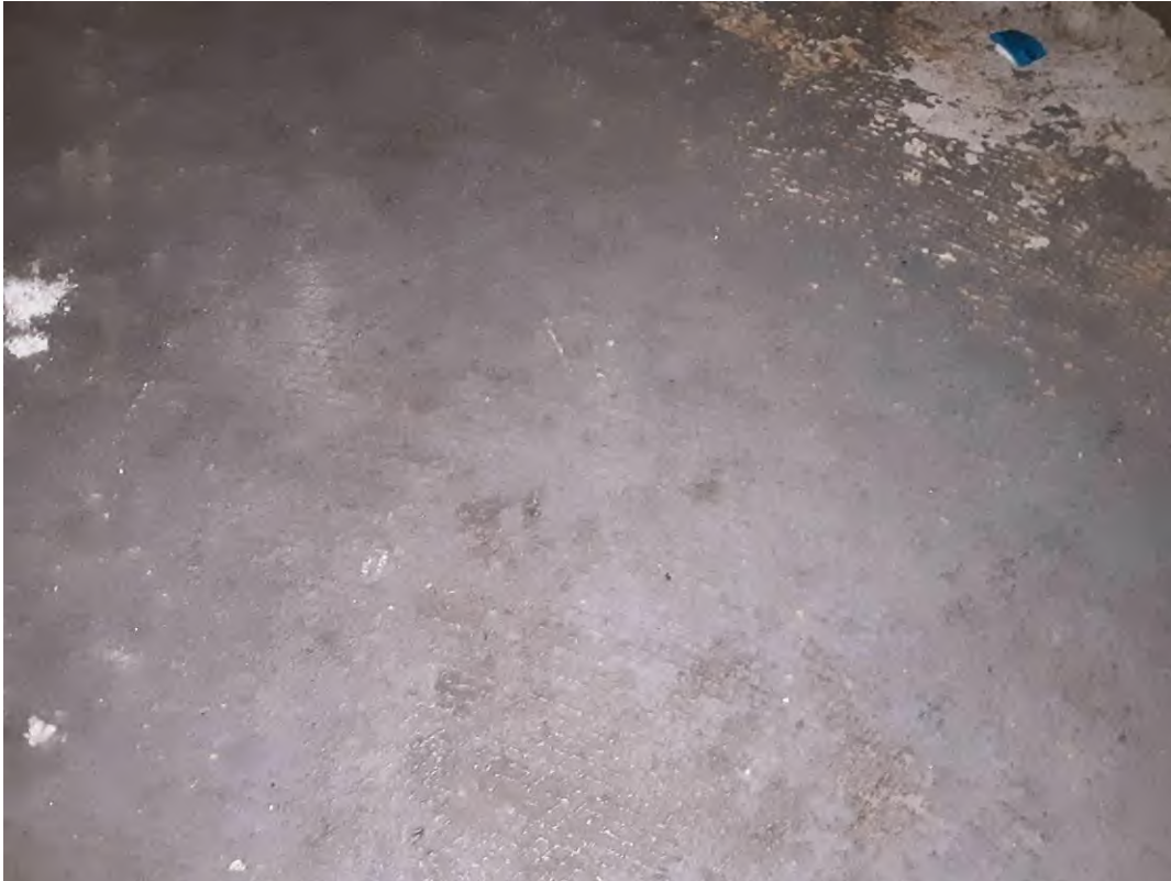
S0058C (None), Floor, All, Mastic, Storage (Location #: 163)
