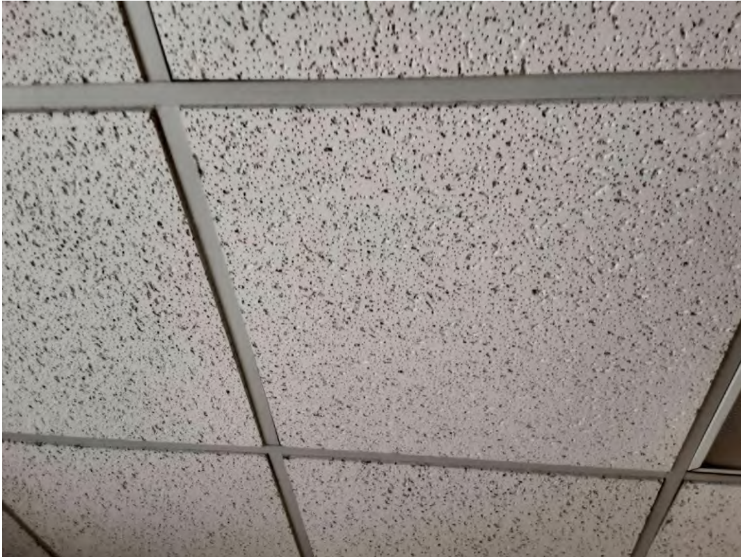
V0000 (None), Ceiling, All, Ceiling Tiles (lay-in), Meeting And Training Room (Location #: 150) Date code 1996
