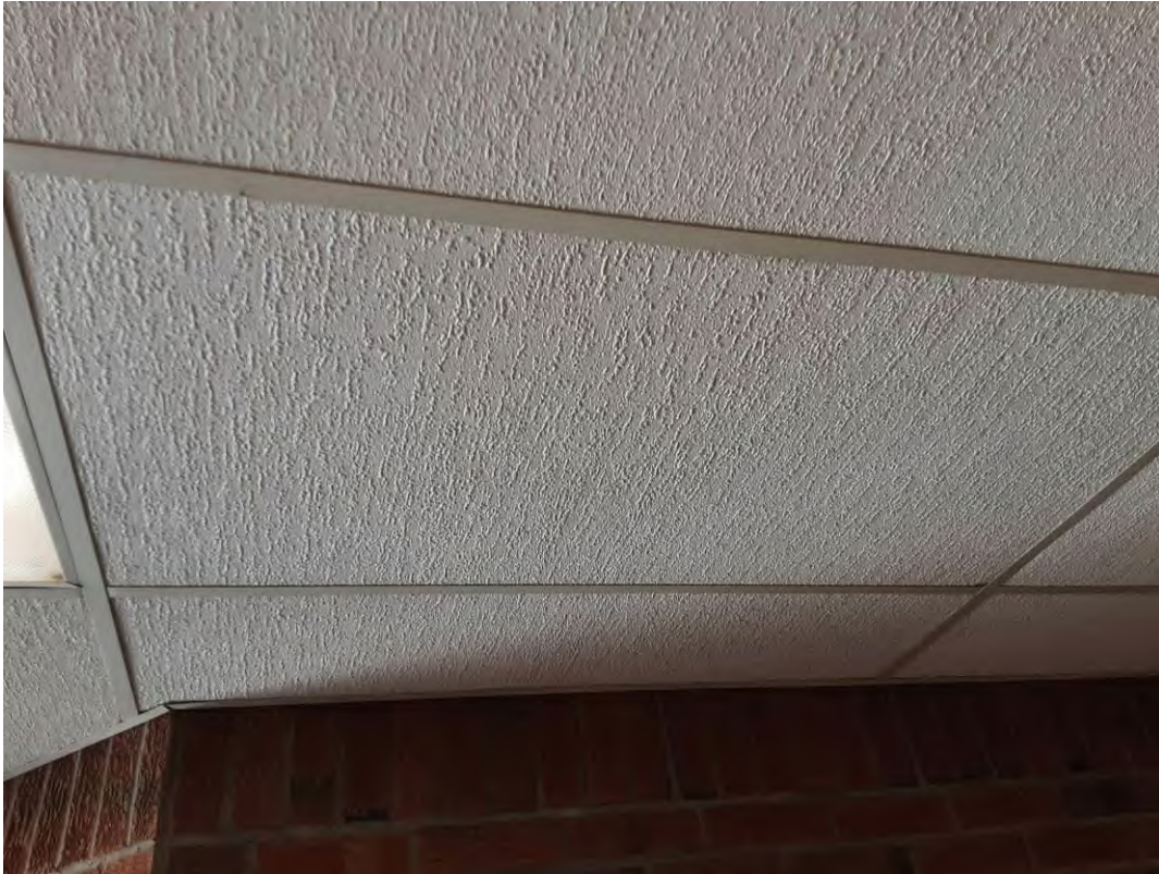
V0000 (None), Ceiling, All, Ceiling Tiles (lay-in), Vestibule (Location #: 3) Fiberglass
