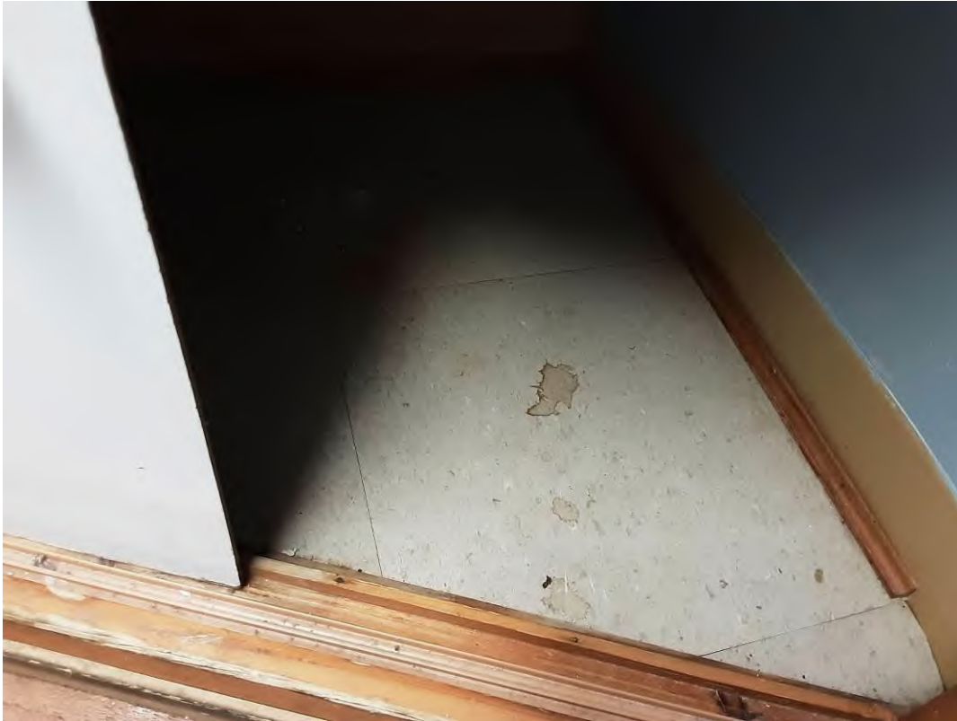
S0021A (None), Floor, Vinyl Floor Tile and Mastic, Tenant Room (Location #: 19) Under washroom millwork
