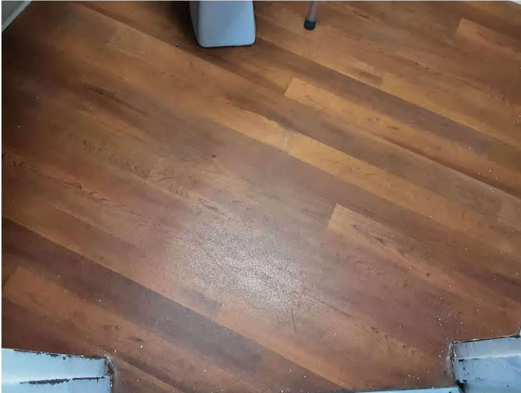
S0018A (None), Floor, Vinyl Sheet Flooring, Tenant Room (Location #: 14)
