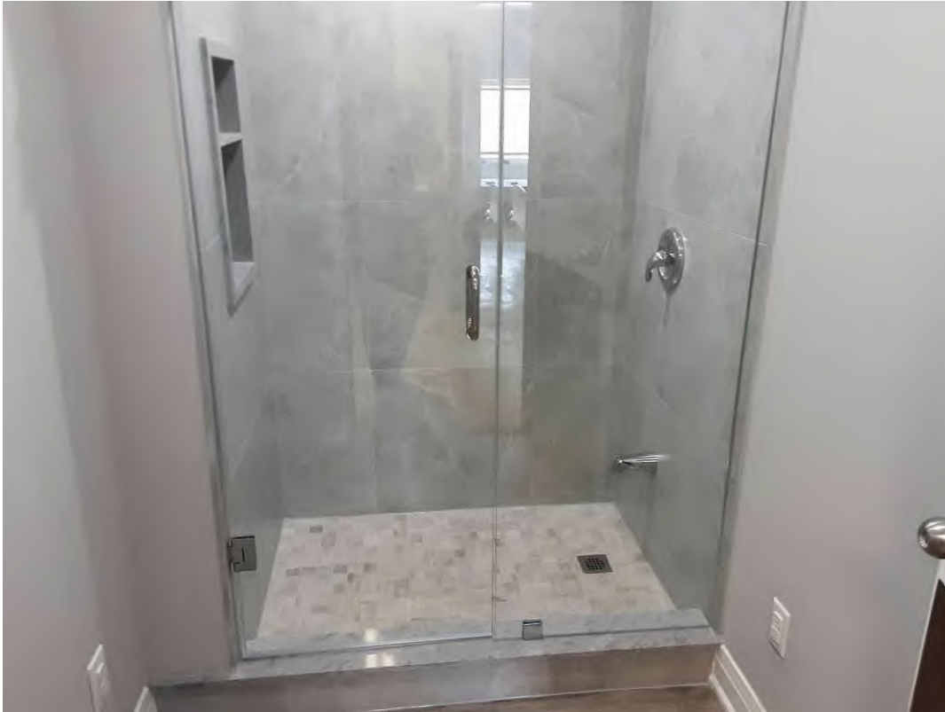
V0000 (None), Wall, Shower Room (Location #: 46)
