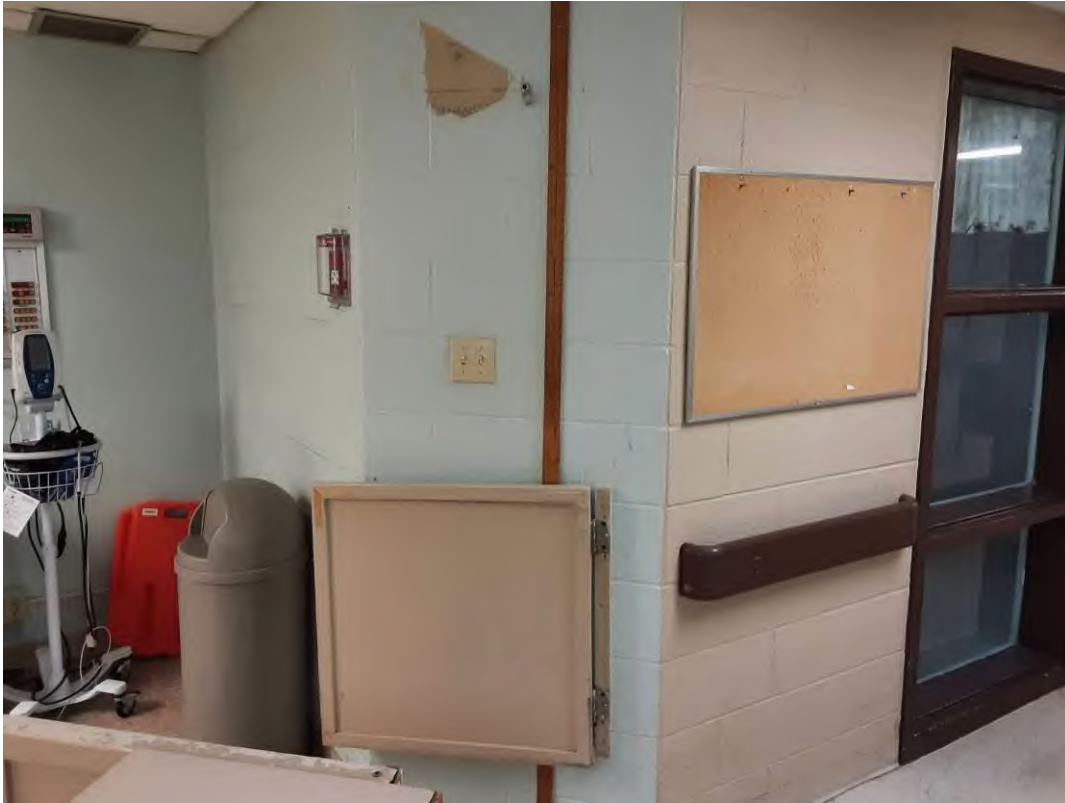
S0007A (None), Wall, Paint, Lobby (Location #: 4)
