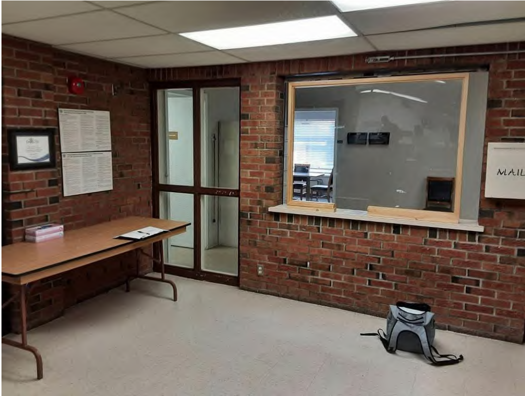
Wall, All, Masonry, Lobby (Location #: 4)
