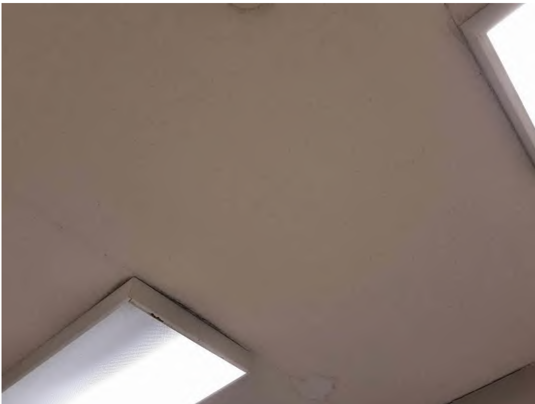
S0008A (None), Ceiling, All, Texture Coat, Main Office (Location #: 5)
