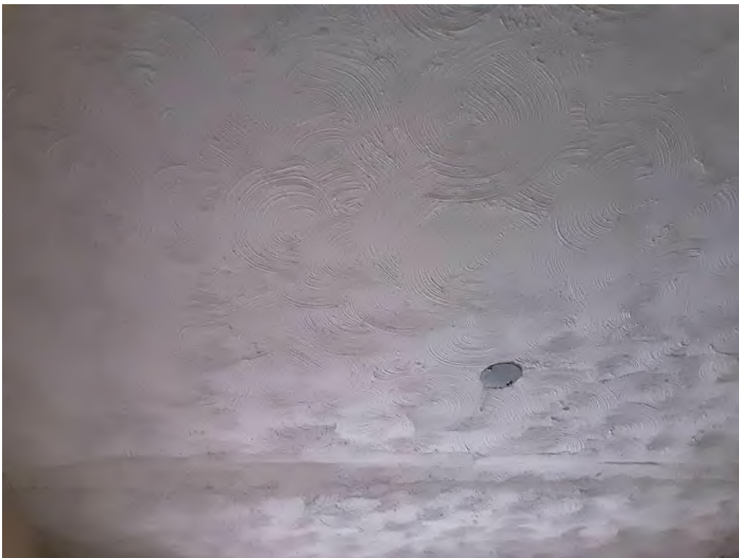
S0064C (None), Ceiling, Texture Coat, Old House - Ground Floor (Location #: 177)
