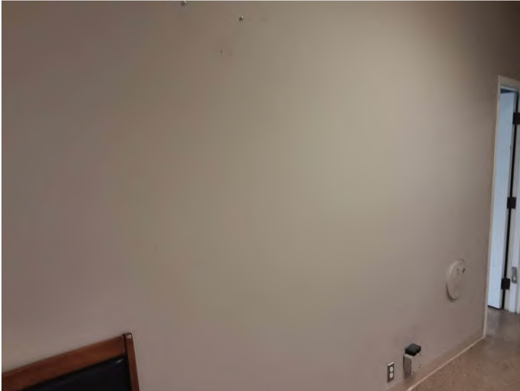
Drywall and joint compound, Light grey paint, L0002, Main Office (Location #: 5)
