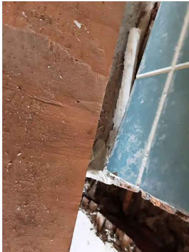
PCB, Old House - 2nd Floor (Location #: 178)
