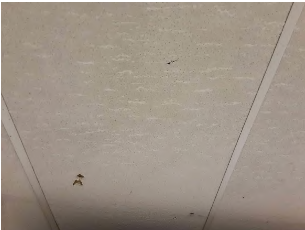
V0000 (None), Ceiling, All, Ceiling Tiles (lay-in), Med Room (Location #: 32) Fiberglass lay-in ceiling tile
