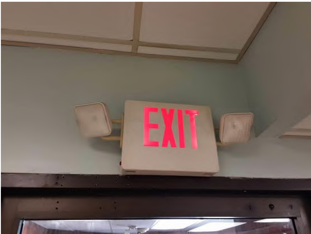
Pb Products, Lobby (Location #: 4)
