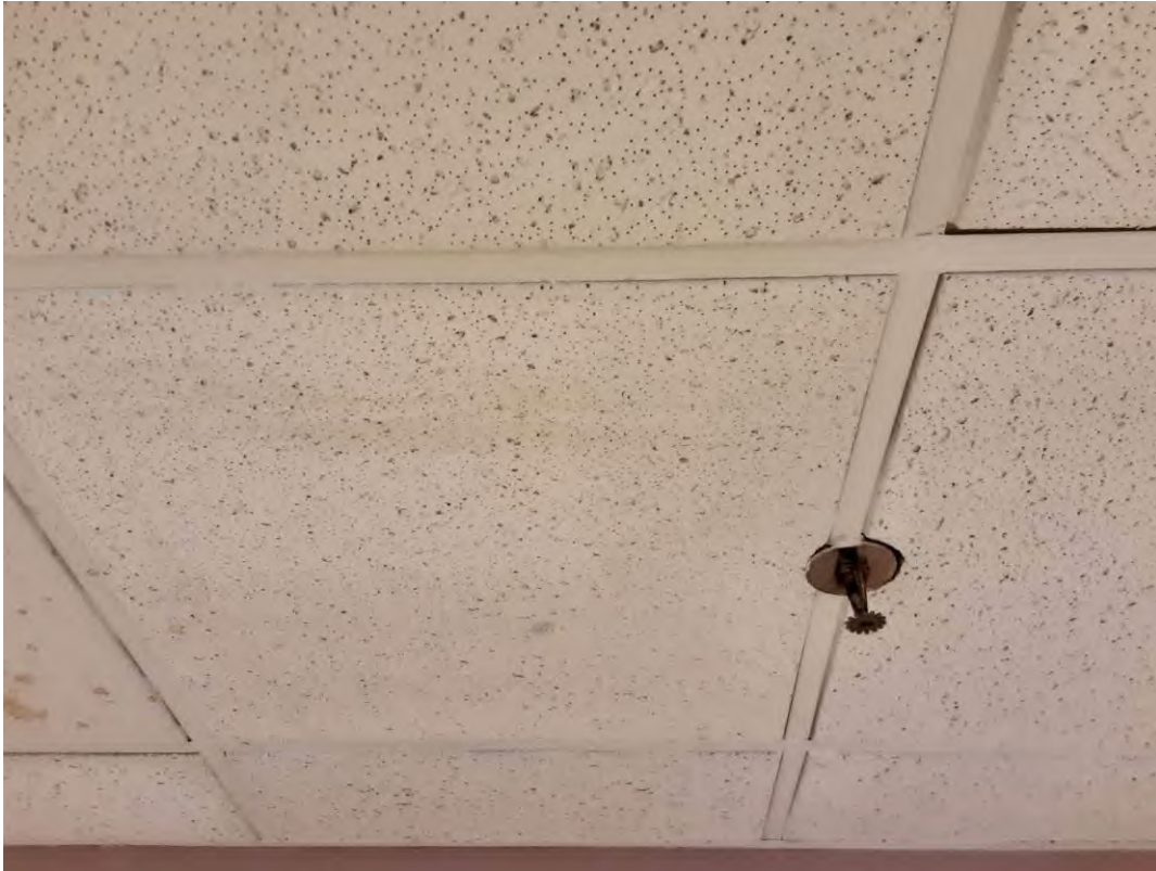
V0000 (None), Ceiling, Ceiling Tiles (lay-in), Dining Room (Location #: 113) Date code 1994
