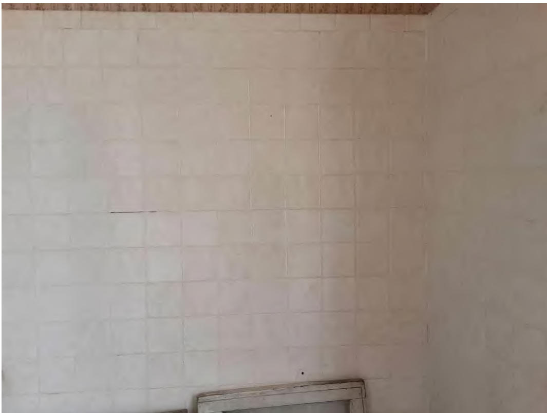
S0068C (None), Wall, Mortar, Old House - 2nd Floor (Location #: 178)
