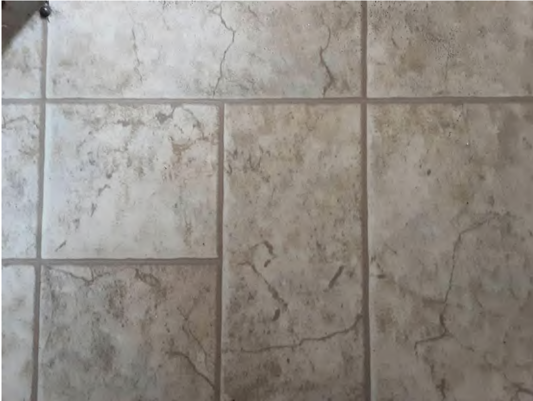
S0037A (None), Floor, Vinyl Sheet Flooring, Tenant Room (Location #: 98) VFT present in sample is S0001
