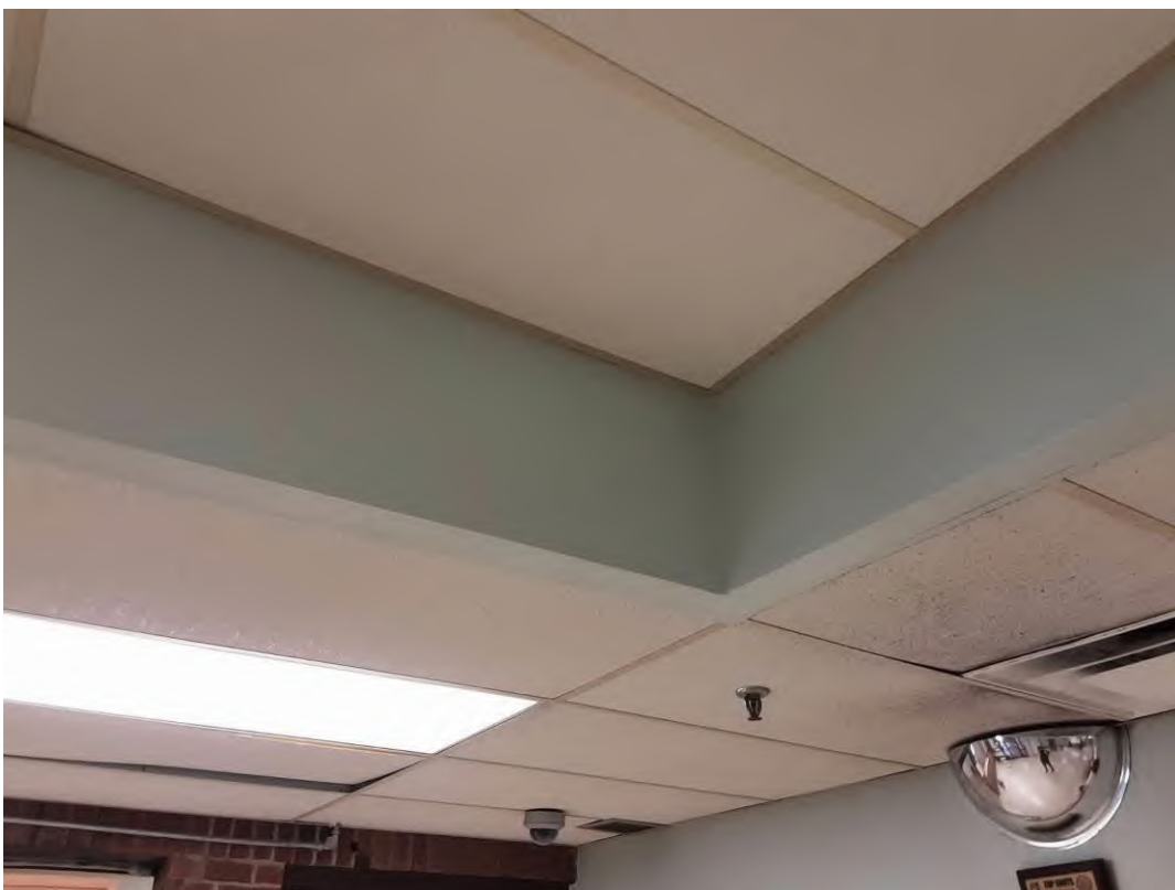
V0000 (None), Ceiling, Drywall (no compound), Lobby (Location #: 4) Mechanically fastened
