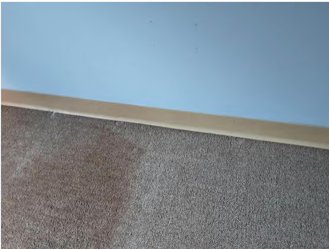
S0052A (None), Wall, Base, Mastic, Medical Supply (Location #: 174)
