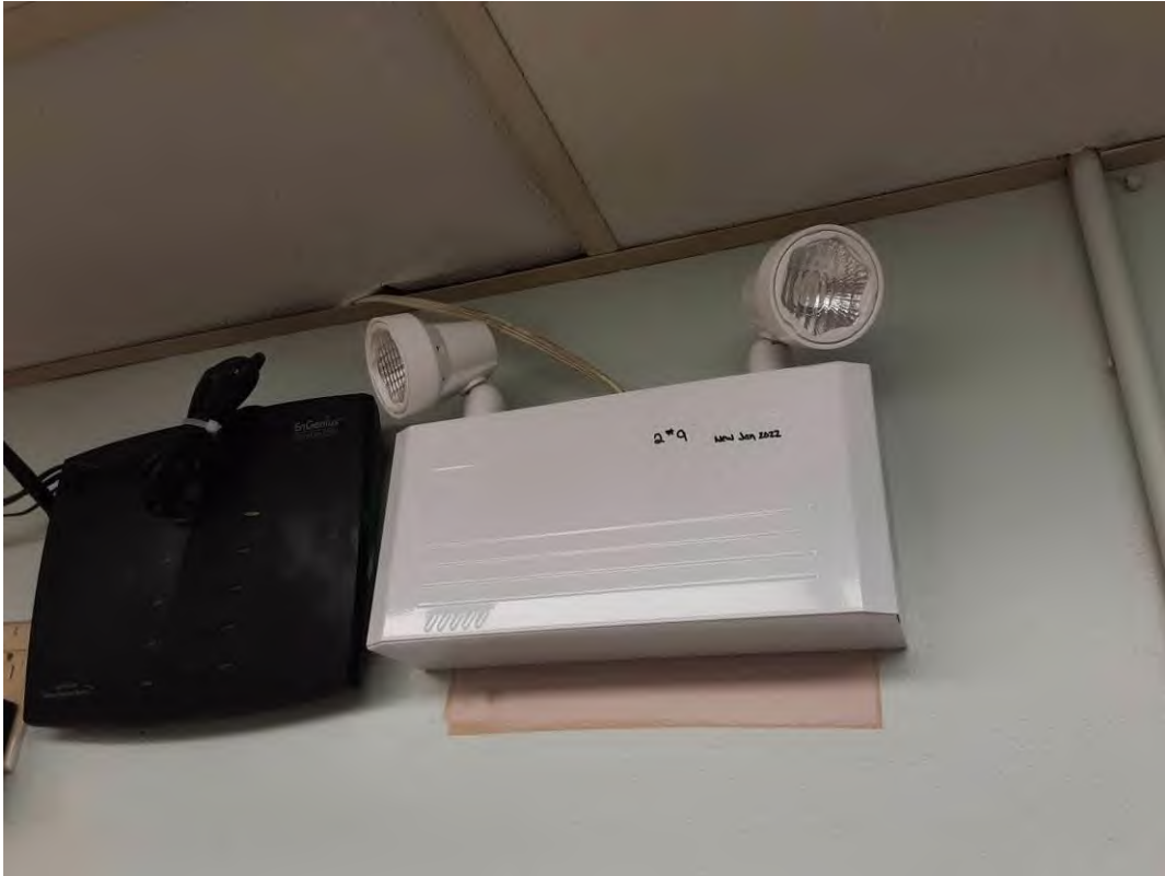
Pb Products, Lobby (Location #: 4)
