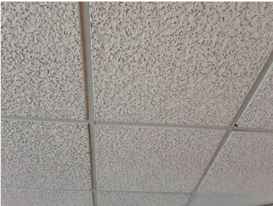
S0013A (None), Ceiling, All, Ceiling Tiles (lay-in), Office (Location #: 10)
