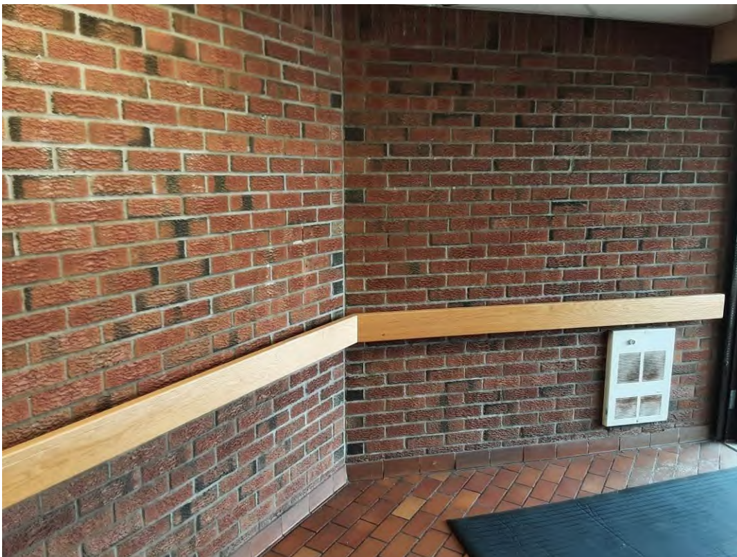
Wall, All, Masonry, Vestibule (Location #: 3)
