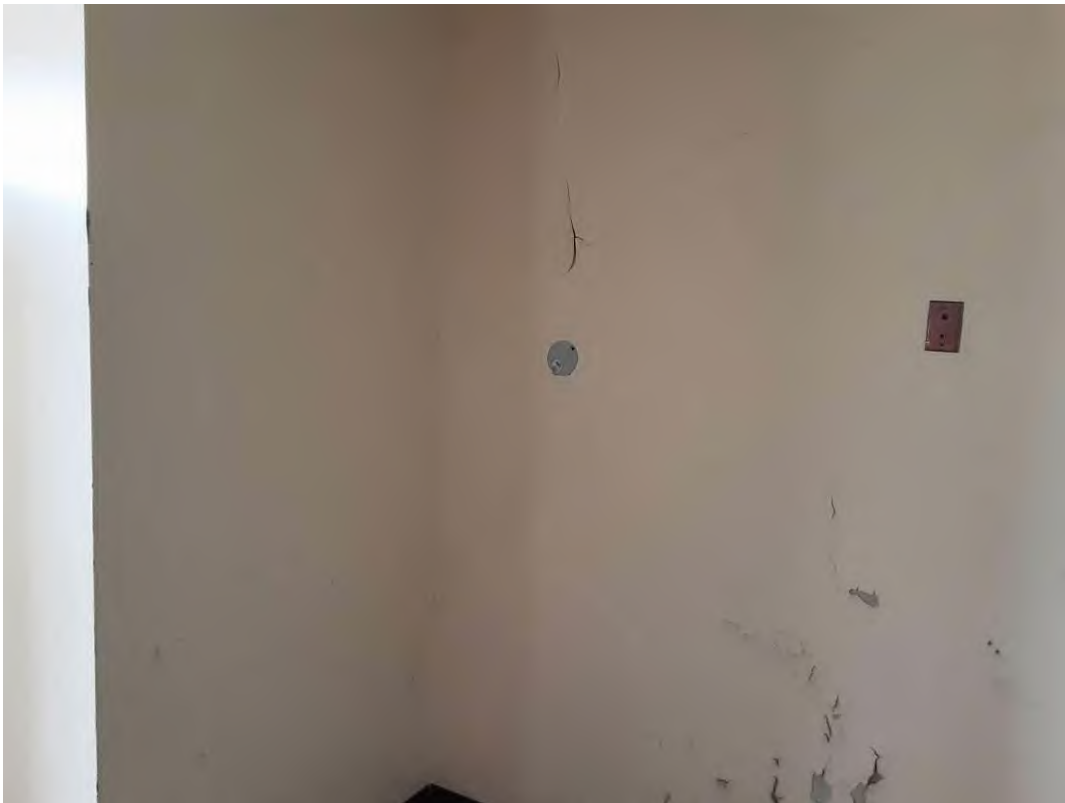
Drywall and joint compound, Off-white, L0016(Lead (High)), Old House - Ground Floor (Location #: 177)
