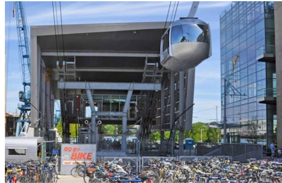
Portland Aerial Tram 2007 Construction
