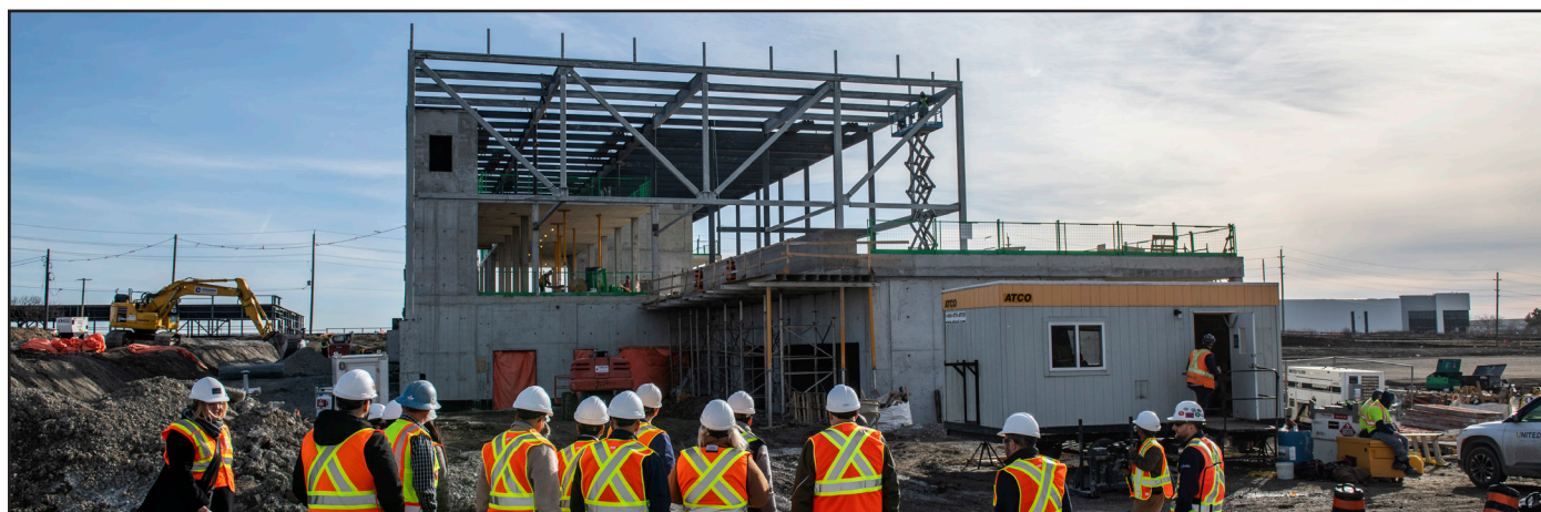
Porsche Experience Construction Site, Pickering
