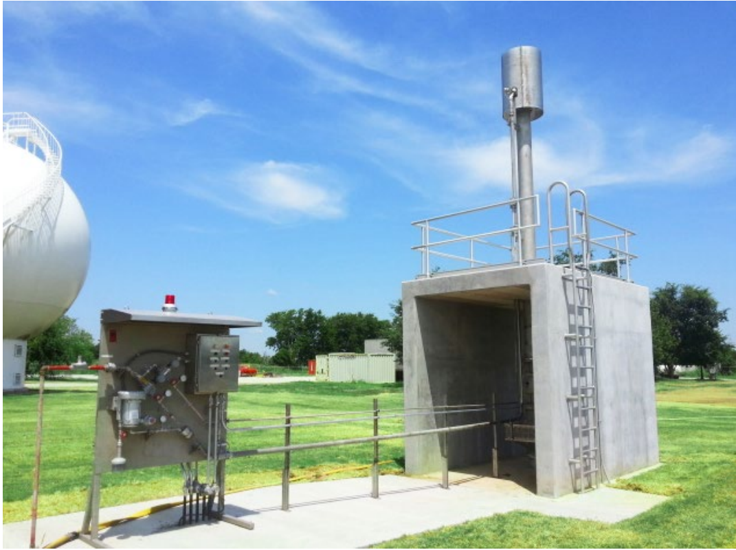
Attachment 1 – Representative Varec Biogas Waste Gas Burner Installation
