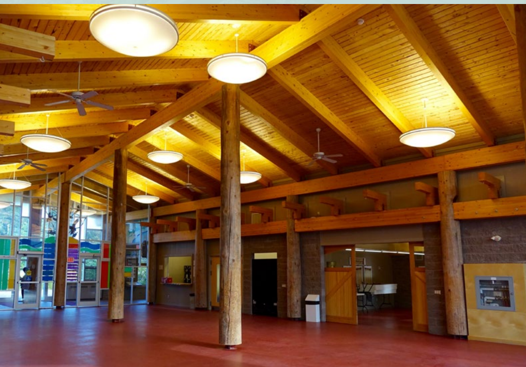
Ganaraska Forest Centre Building Interior, Clarington
