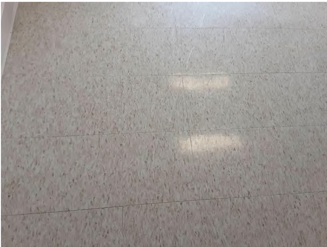
S0070A (None), Floor, Vinyl Floor Tile and Mastic, Office (Location #: 161)
