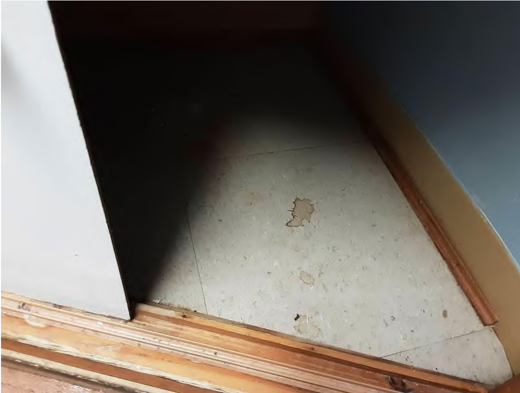
S0021A (None), Floor, Vinyl Floor Tile and Mastic, Tenant Room (Location #: 19) Under washroom millwork
