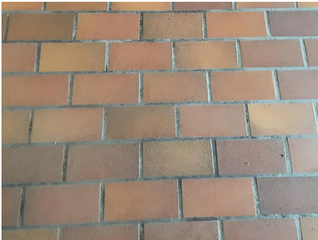
S0079A (Confirmed Asbestos), Floor, Mortar, under 2" x 6" red faux brick ceramic tile, Vestibule (Location #: 116)
