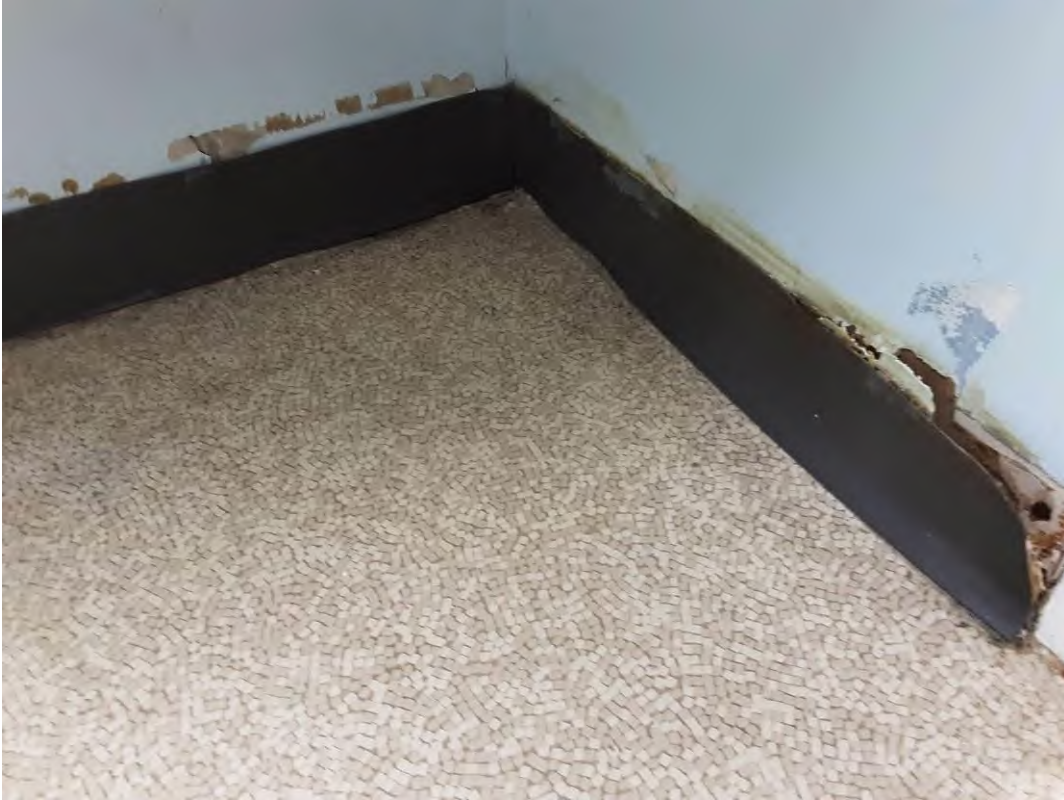
S0014A (None), Wall, Base, Adhesive/mastic, Visitors Washroom (Location #: 13)
