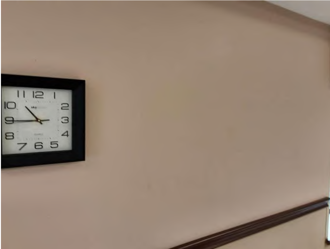
Drywall and joint compound, Pink paint, L0010, Dining Room (Location #: 58)
