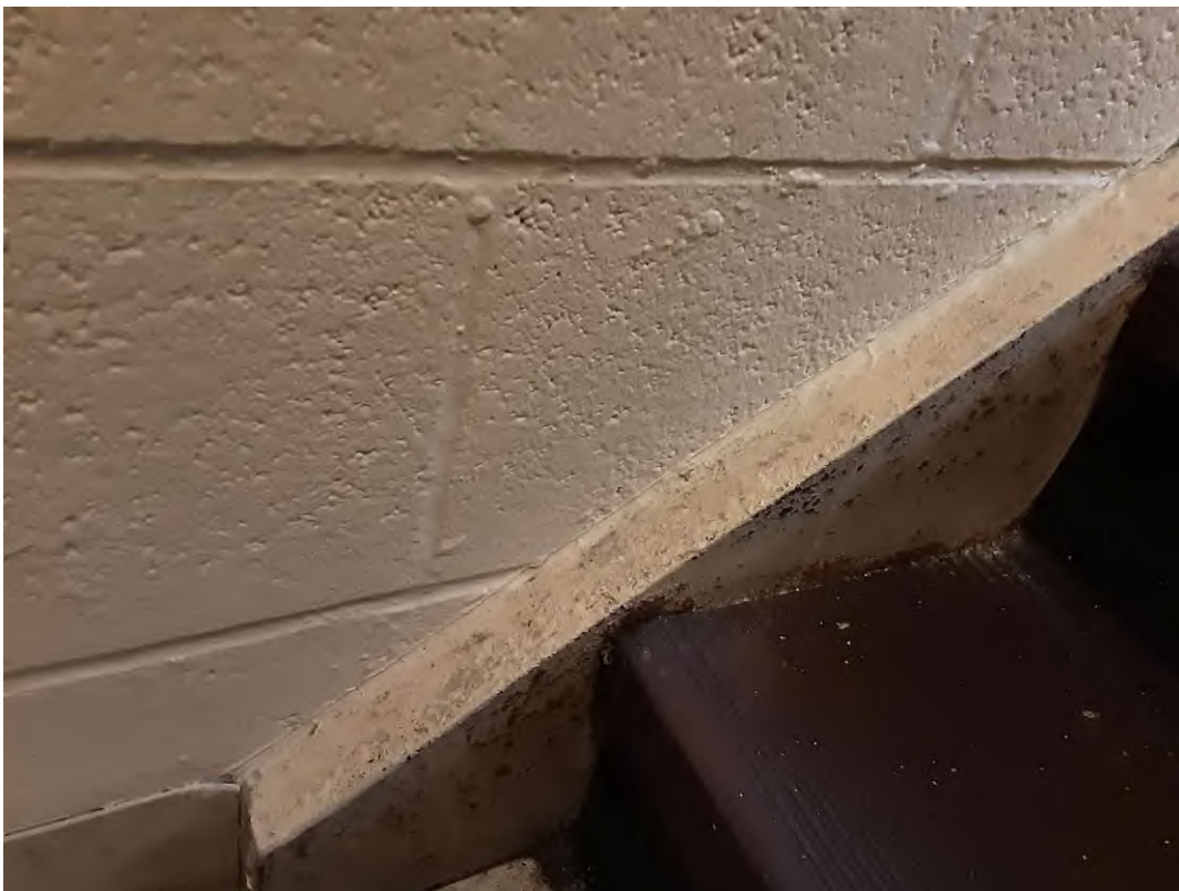
S0047A (None), Structure, Caulking, South Stairwell (Location #: 143)
