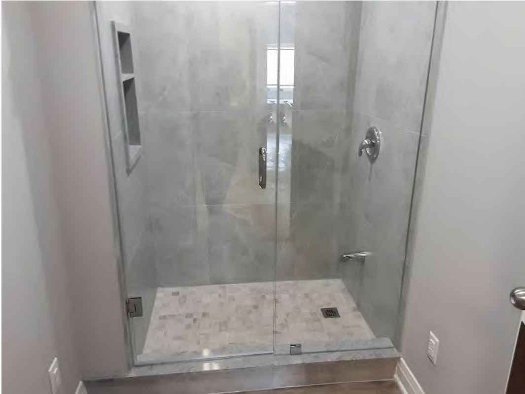
V0000 (None), Wall, Shower Room (Location #: 46)
