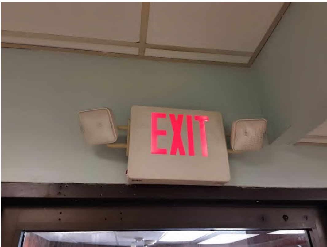
Pb Products, Lobby (Location #: 4)
