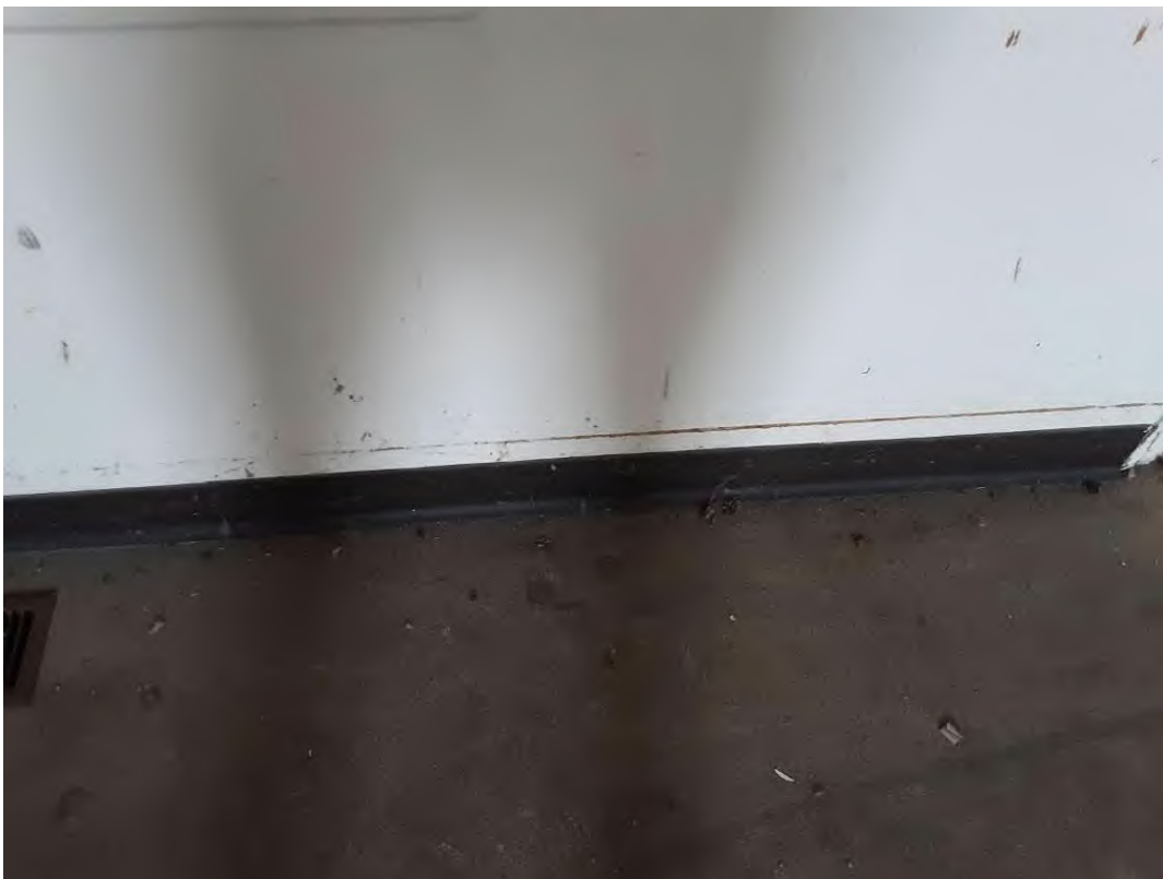
S0061C (None), Wall, Base, Adhesive/mastic, Old House - Ground Floor (Location #: 177)
