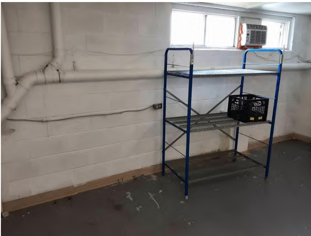
V9000 (Confirmed Asbestos), Piping, Rain Water Leader, Cement Product, Dietary Storage (Location #: 130)
