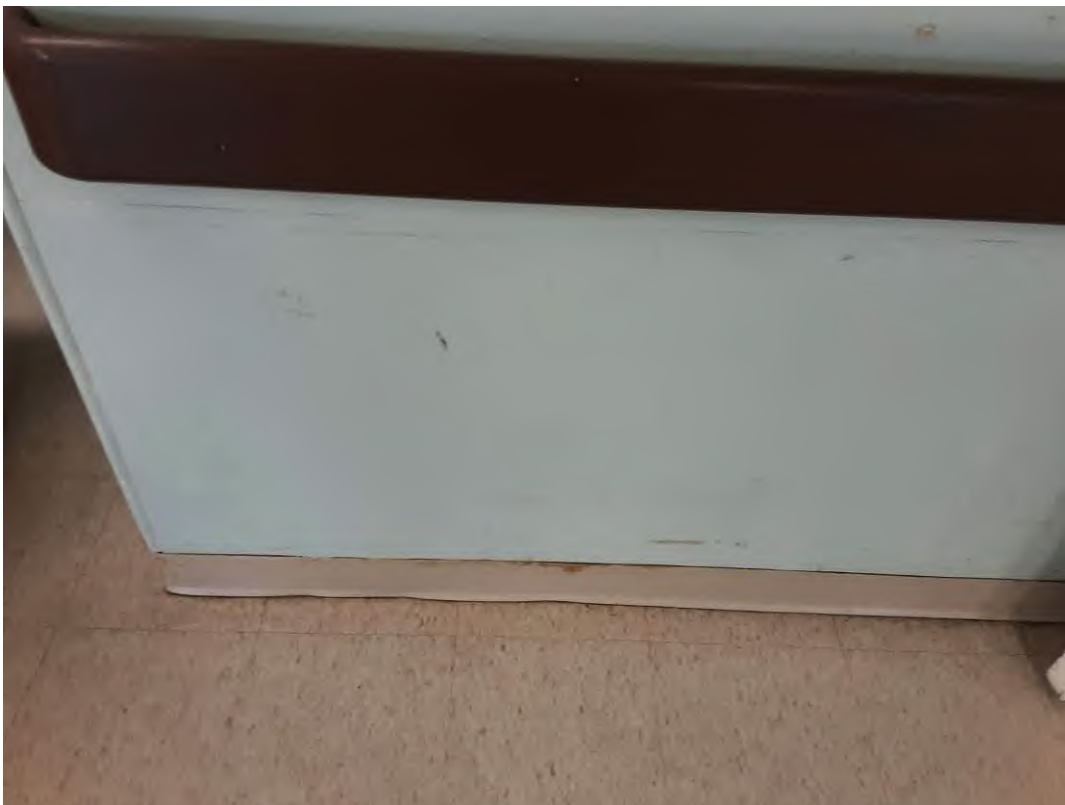
S0002A (None), Wall, Base, Adhesive/mastic, Lobby (Location #: 4)
