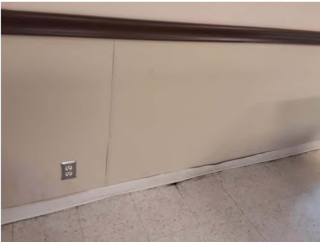
S0031A (None), Wall, Base, Wall covering, Dining Room (Location #: 58)
