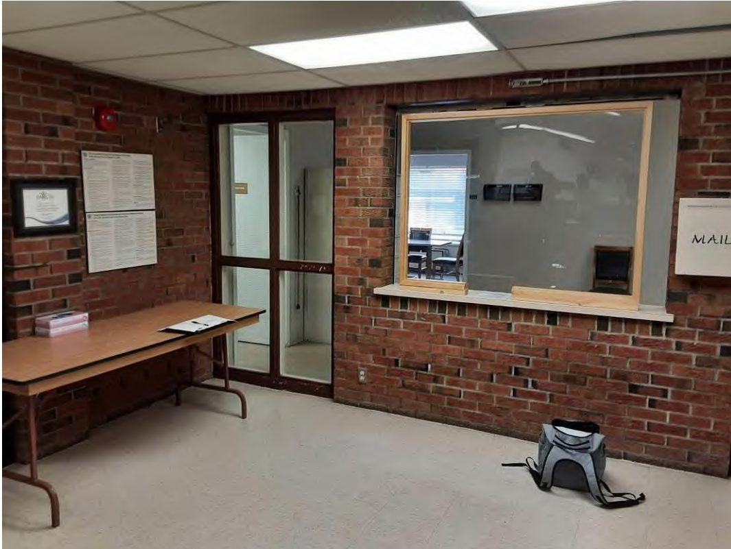
Wall, All, Masonry, Lobby (Location #: 4)
