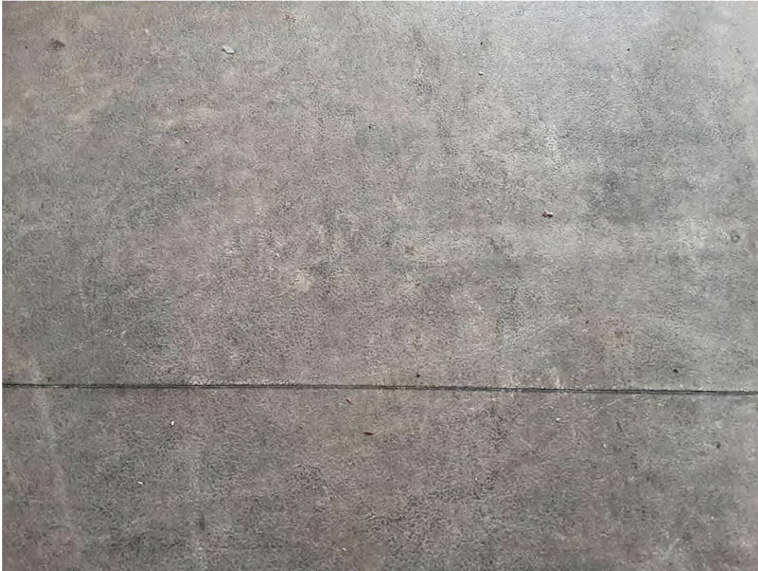
S0060A (None), Floor, Vinyl Sheet Flooring, Old House - Ground Floor (Location #: 177)
