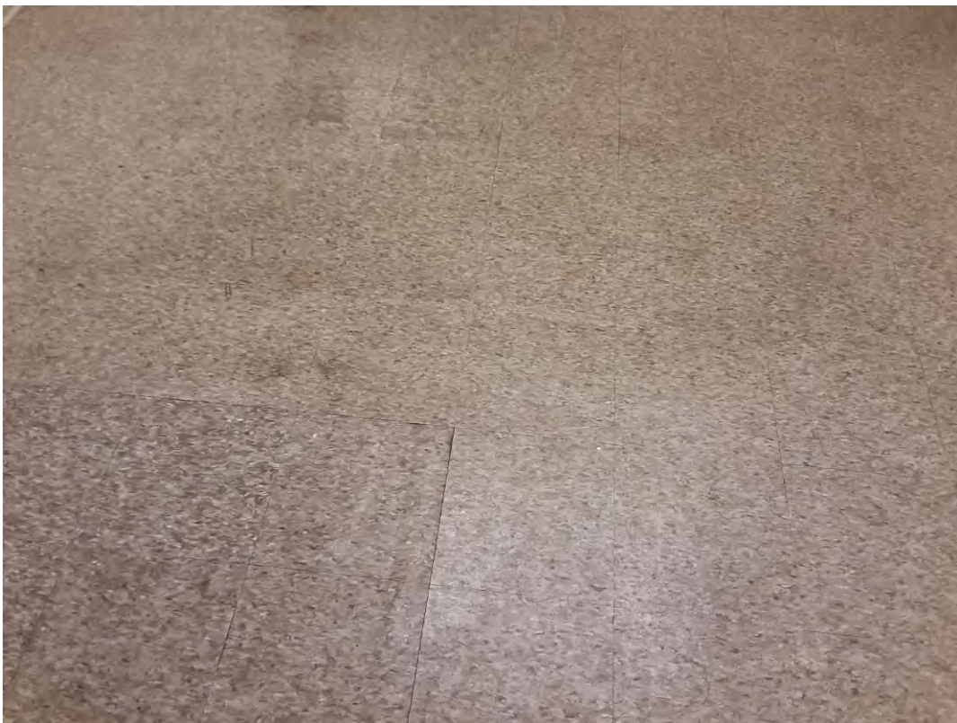
V0003 (None), Floor, Vinyl Floor Tile and Mastic, Main Office (Location #: 5)
