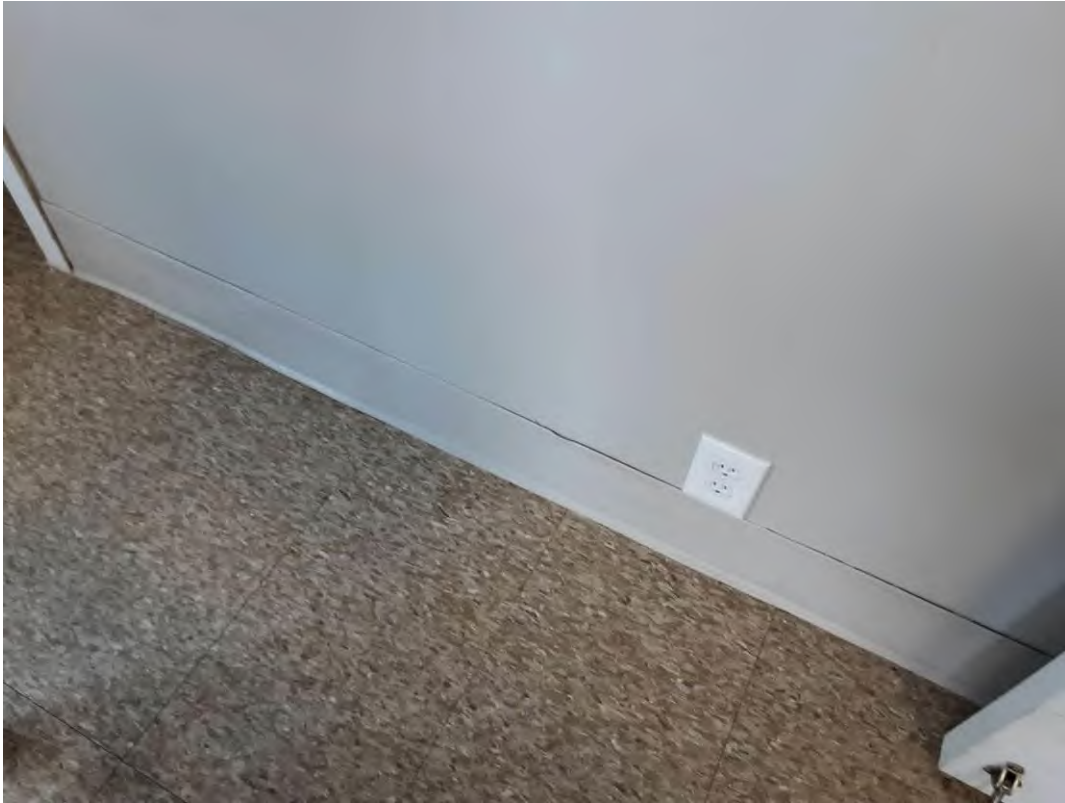
S0010A (None), Wall, Base, Adhesive/mastic, Meeting Room (Location #: 7)
