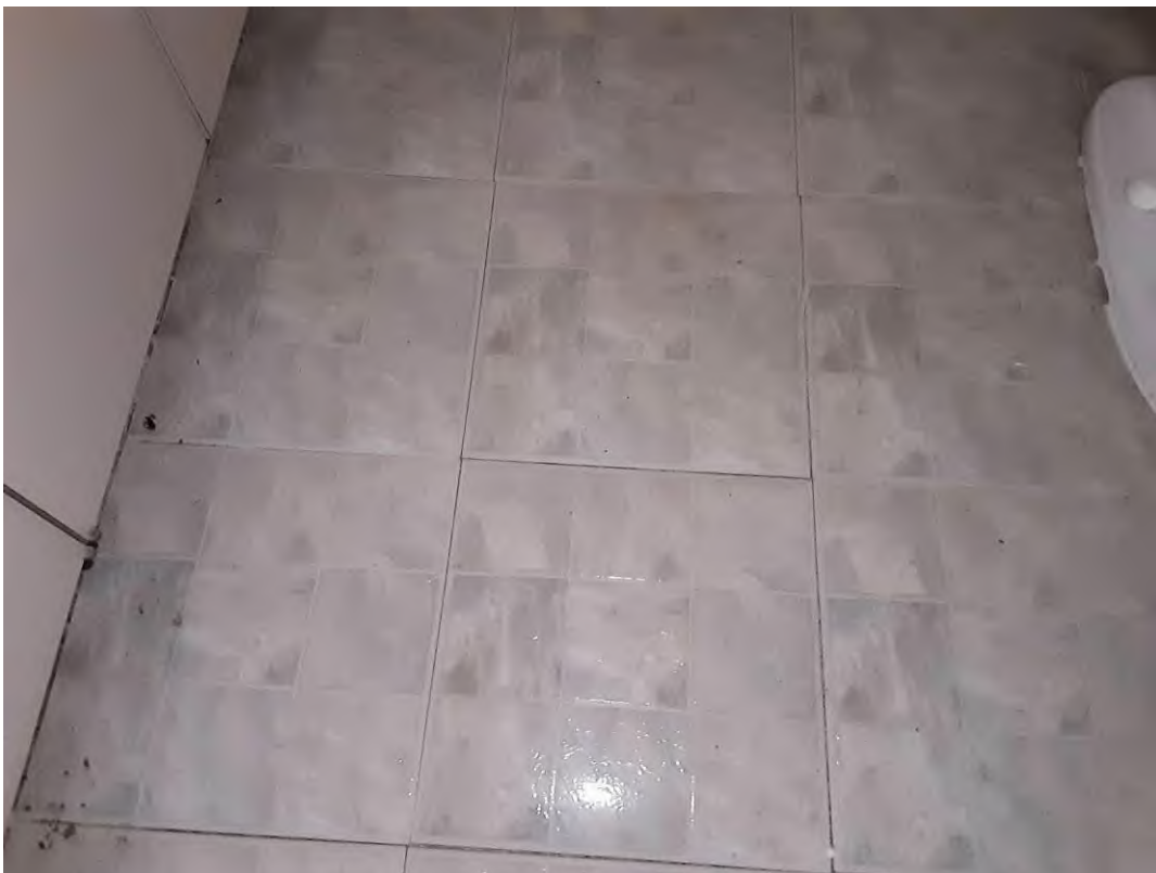
S0054A (Confirmed Asbestos), Floor, Vinyl Floor Tile and Mastic, Records (Location #: 171)
