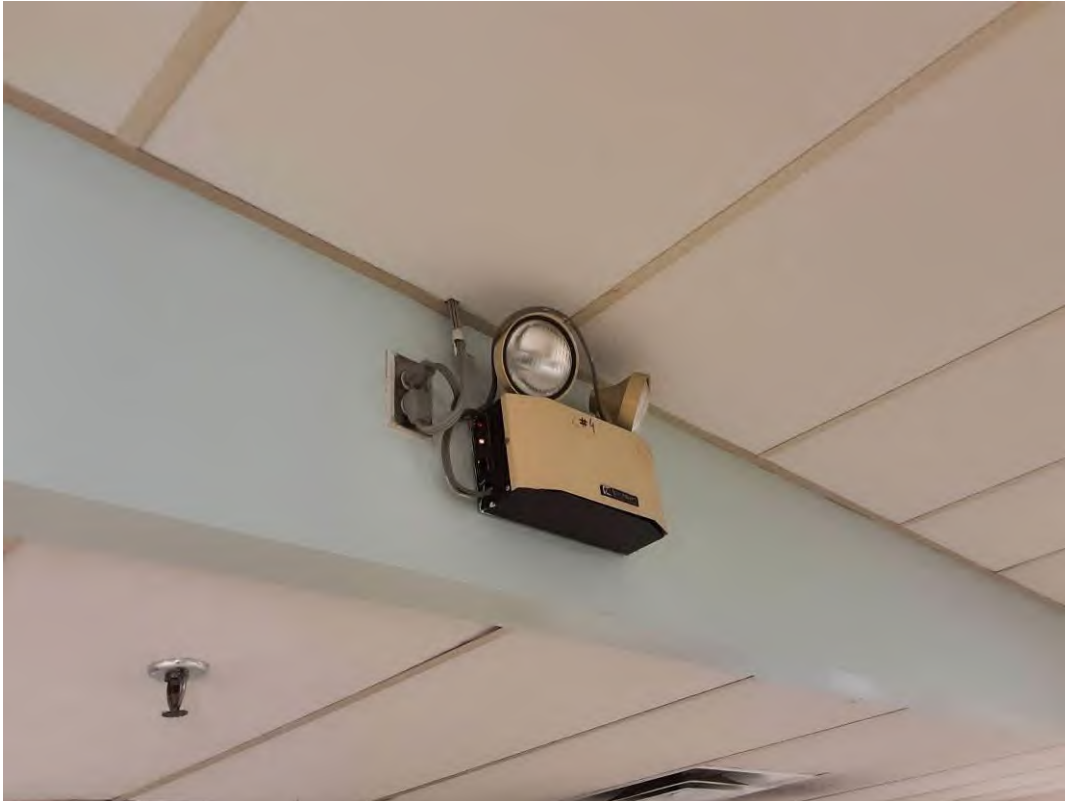
Pb Products, Lobby (Location #: 4)
