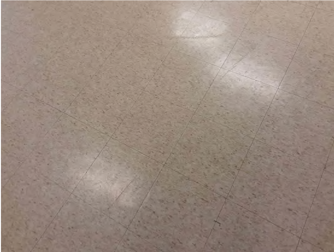
S0001A (None), Floor, All, Vinyl Floor Tile and Mastic, Lobby (Location #: 4)
