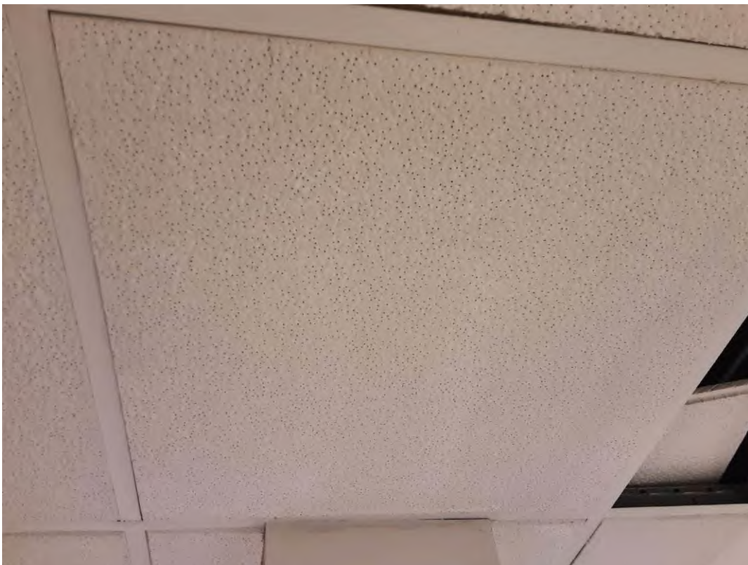
V0000 (None), Ceiling, Ceiling Tiles (lay-in), Dining Room (Location #: 113) Date code 2004
