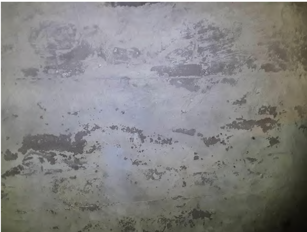
S0041A (None), Wall, All, Plaster, Old House - Basement (Location #: 135)
