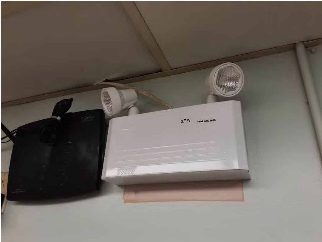
Pb Products, Lobby (Location #: 4)
