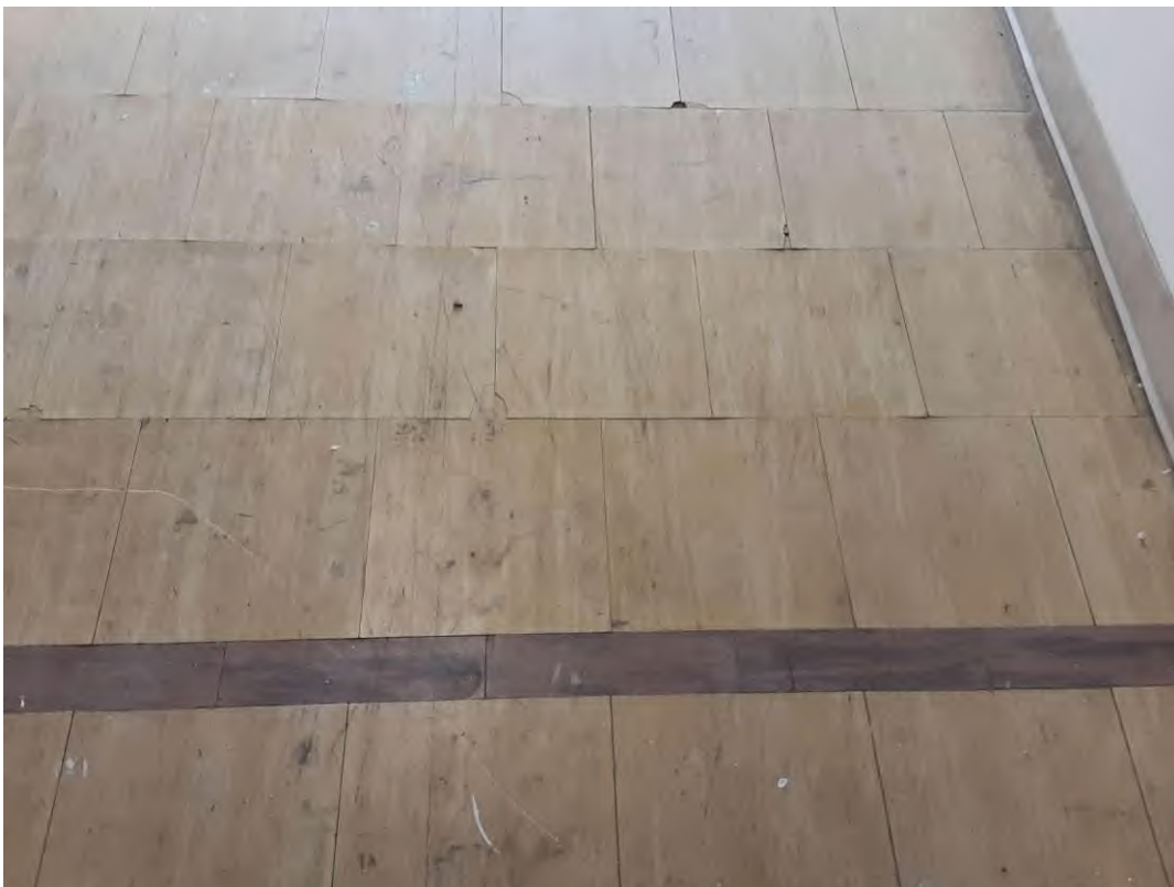
S0059C (Confirmed Asbestos), Floor, All, Vinyl Floor Tile and Mastic, Foyer (Location #: 149)
