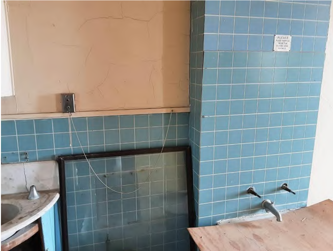
V0000 (None), Wall, Fibrous Board, Old House - 2nd Floor (Location #: 178)
