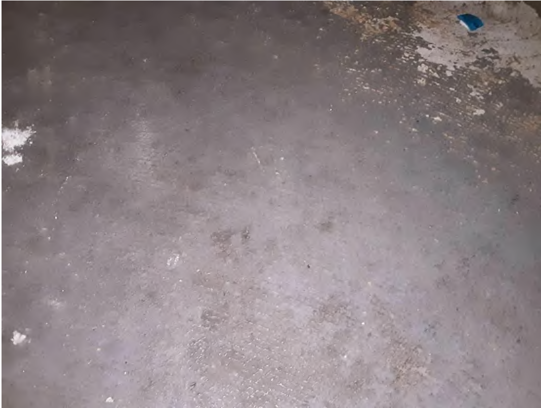
S0058C (None), Floor, All, Mastic, Storage (Location #: 163)
