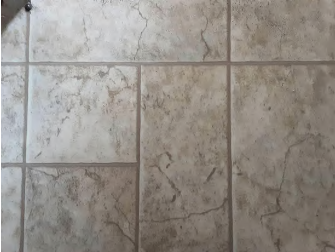
S0037A (None), Floor, Vinyl Sheet Flooring, Tenant Room (Location #: 98) VFT present in sample is S0001
