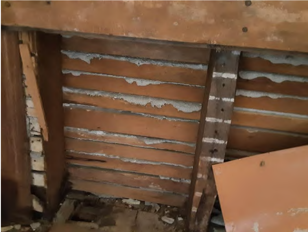
S0041C (None), Wall, All, Plaster, Old House - Ground Floor (Location #: 177)
