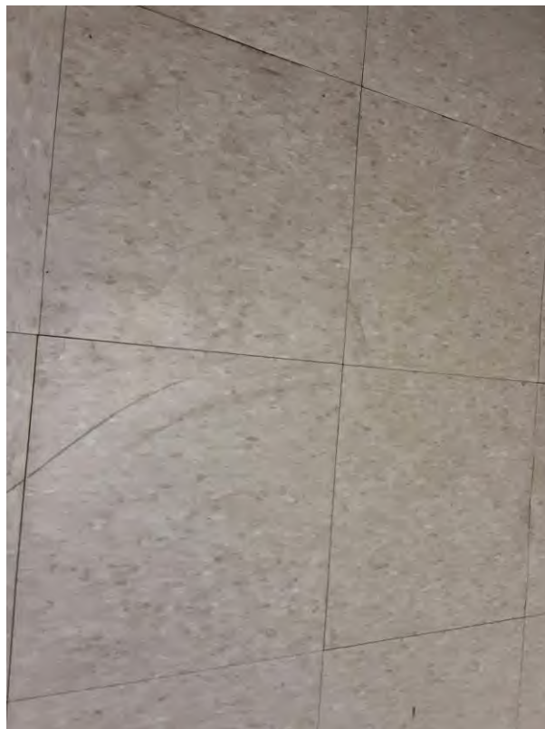
S0022A (None), Floor, Vinyl Sheet Flooring, Tenant Room (Location #: 25)
