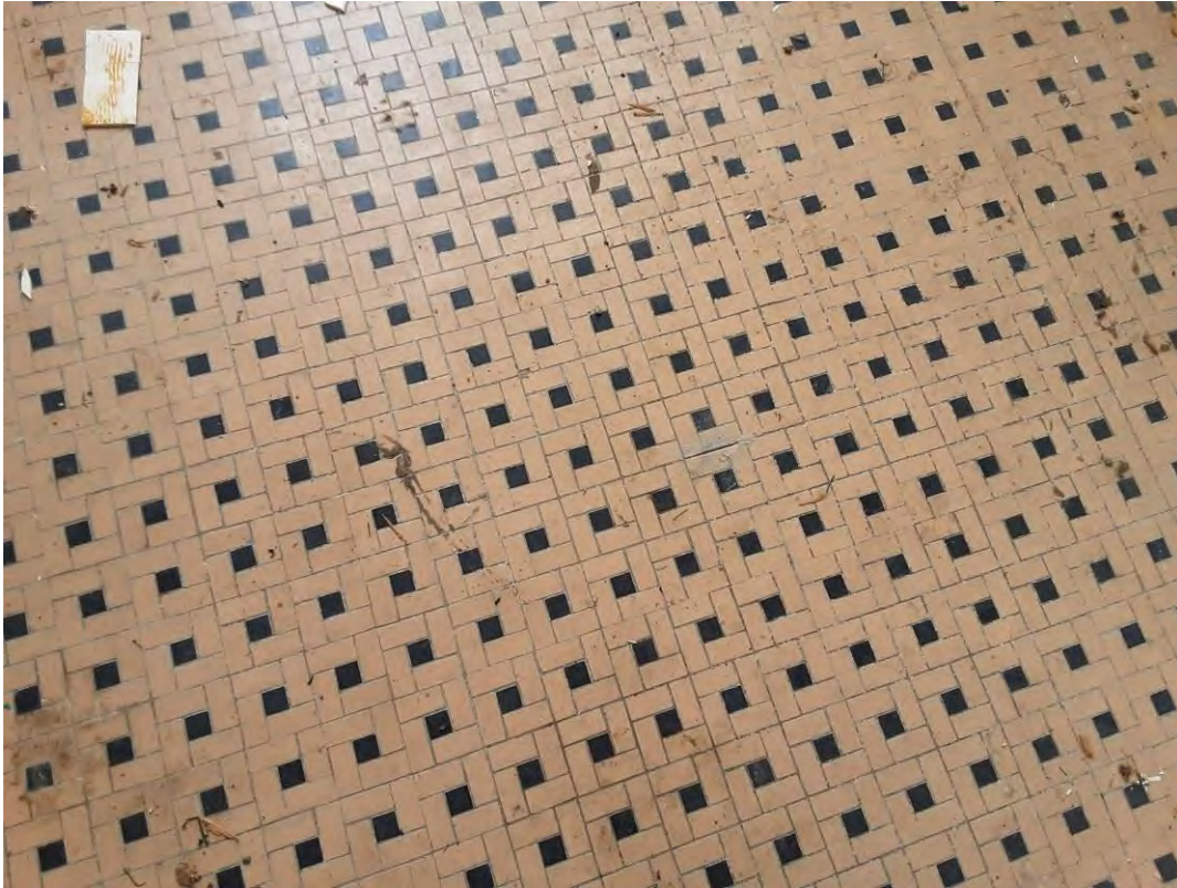
S0067C (None), Floor, Mortar, Old House - 2nd Floor (Location #: 178)
