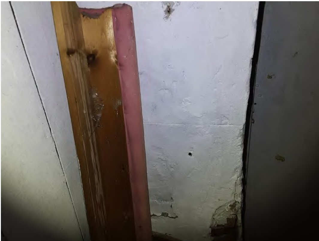
Plaster, White paint on plaster, L0012, Old House - Basement (Location #: 135)
