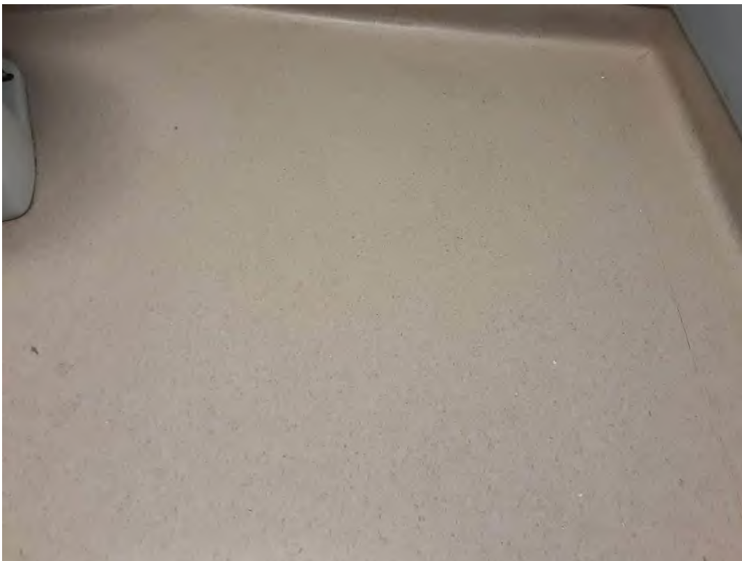
S0019A (None), Floor, Vinyl Sheet Flooring, Tenant Room (Location #: 16)
