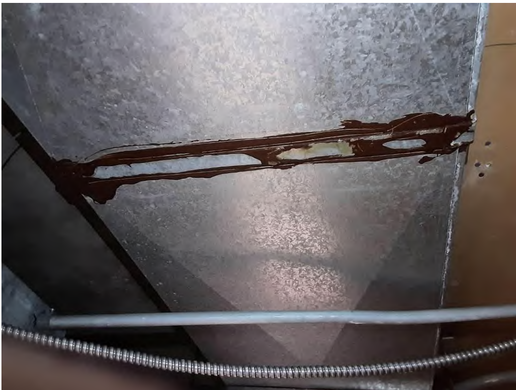
S0029A (None), Duct, Caulking, North Corridor (Location #: 57)
