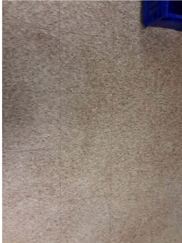
S0003A (None), Floor, Vinyl Floor Tile and Mastic, Lobby (Location #: 4)
