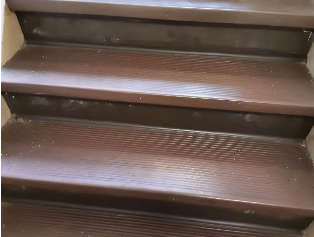
S0048A (None), Floor, Non-slip Flooring, South Stairwell (Location #: 143)
