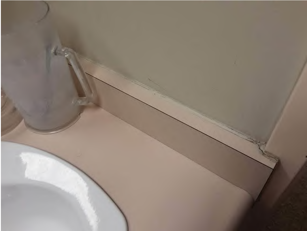
S0012A (None), Other, Caulking, Office (Location #: 9)
