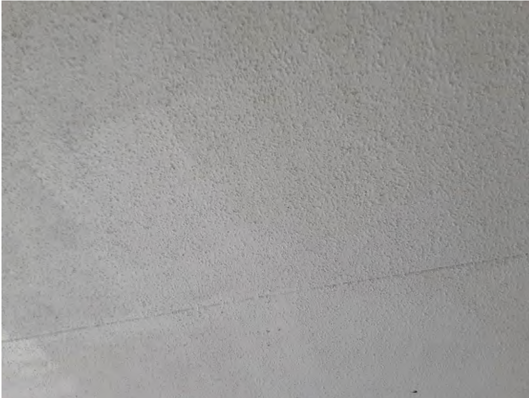
S0051A (None), Ceiling, All, Texture Coat, Medical Supply (Location #: 174)
