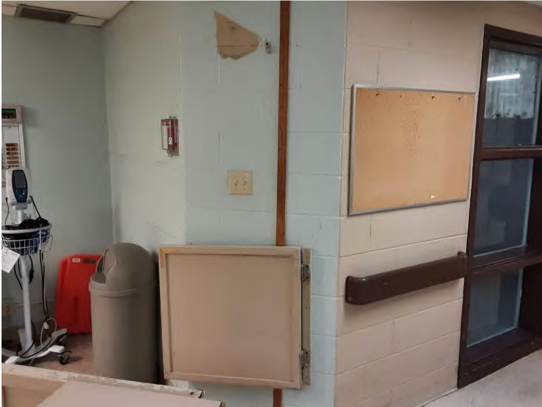
S0007A (None), Wall, Paint, Lobby (Location #: 4)
