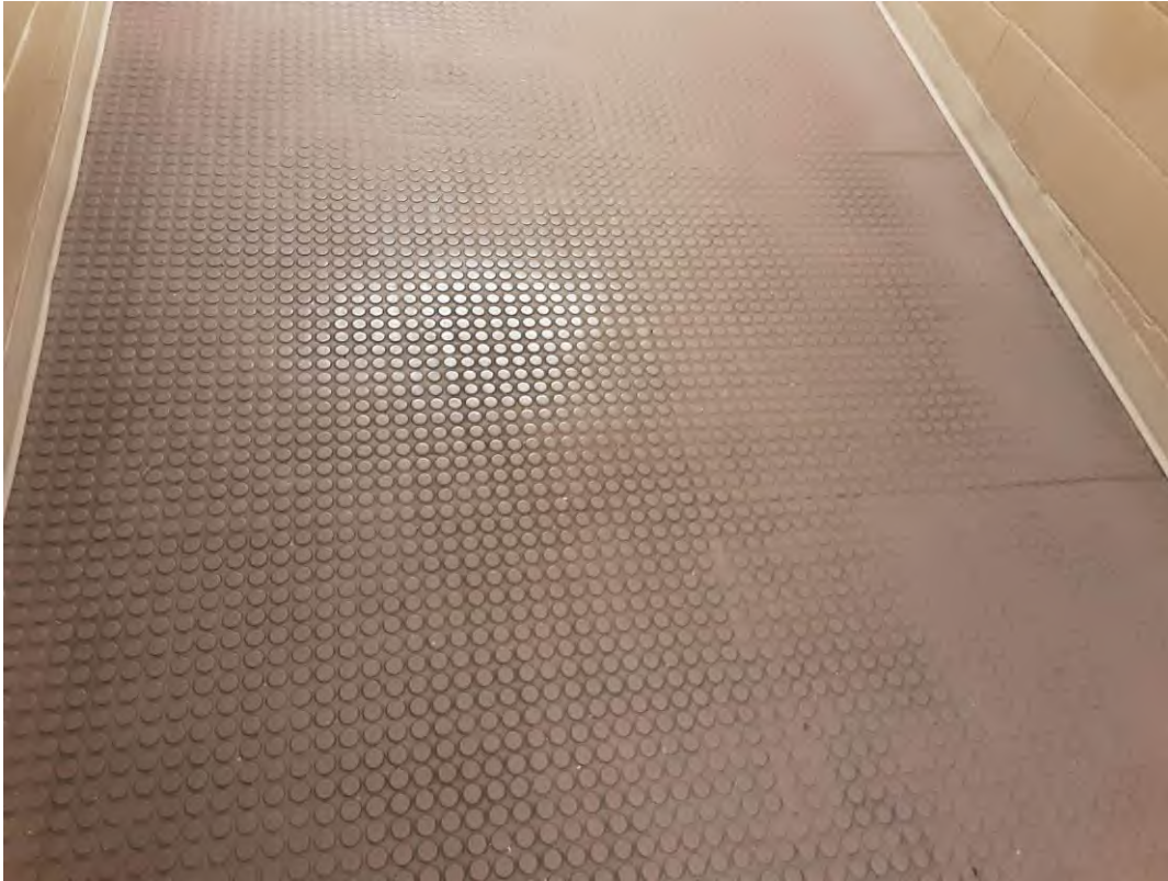
S0046A (Confirmed Asbestos), Floor, Non-slip Flooring, North Corridor (Location #: 142)
