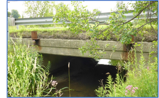
Central St. Over Mitchell Creek Tributary Bridge
