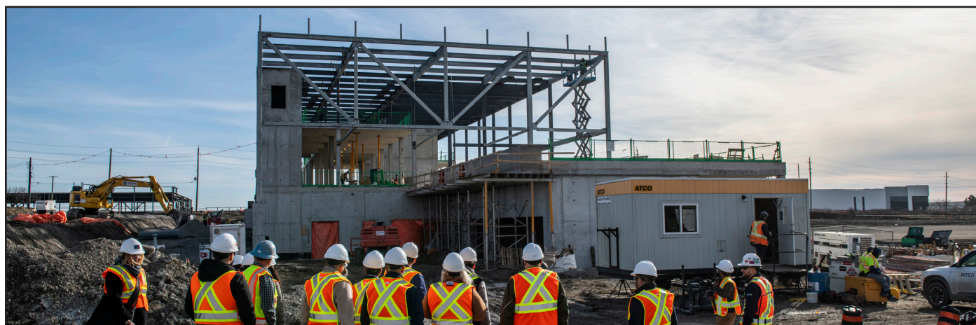
Porsche Experience Construction Site, Pickering
