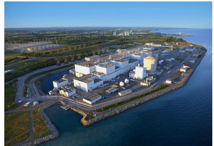
Darlington Nuclear Generating Station Source: OPG
