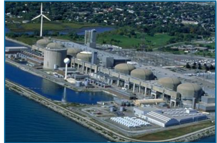
Pickering Nuclear Generating Station Image source: OPG
