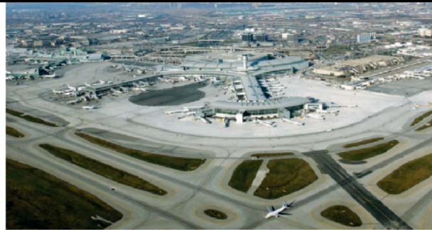
Terminal Apron Areas and Dual Taxiway System
