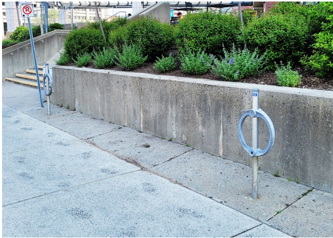
Parallel rack configurations work best in constrained areas
