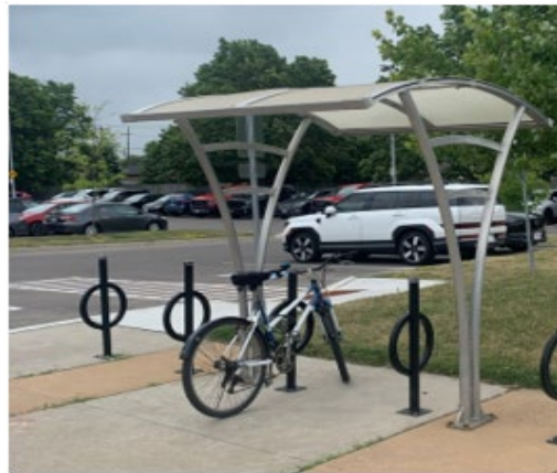
Covered post-and-ring racks
